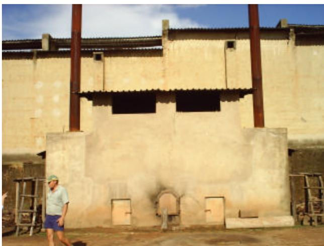
In addition to the traditional method, Ralph Henderson also operates 2 improved curing barns. The curing barn on the left uses an air-to-air heat exchanger to heat multiple barns with a single combustion chamber. This combustion chamber (approx dimensions - 4 m by 3m by 3m) is used to heat a large metal plate and series of metal tubes. A fan drives air from the outside, through these pipes, and over the plate and into 5 separate curing
