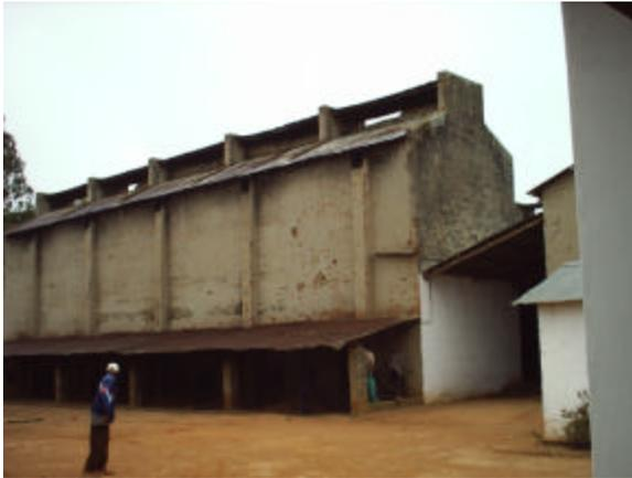
Three types of curing barns are used in Malawi, but **most of the tobacco is cured in traditional barns** similar to the one shown in the photo on left. In the traditional barn there are 5 drying rooms that are fired with 5 separate wood combustion chambers. The 5 chimneys that correlate to the combustion chambers are visible in the photo.
