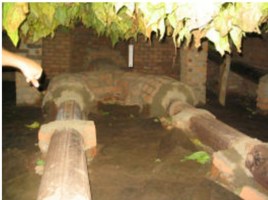
This air is then heated by the exposed chimney pipe that snakes around the bottom of the barn. This hot dry air whisks moisture from the tobacco that is then vented through an adjustable gap in the ceiling of the barn.
