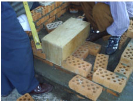
A removable wooden mould is used to construct the combustion chamber. The mould is designed to create a ledge that will support the legless metal wood shelf.
