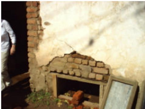
The heat transfer mechanism is very simplistic. Cold air is drawn through 4 small openings at the bottom of the barn (1 of these is shown in photo left).
