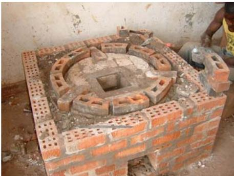
Note the white insulated bricks that are encircled by the curved (non insulated) Kajansi Bricks. Ideally these curved bricks would be insulative as well but strength is a more important consideration than insulation in the circular bricks
