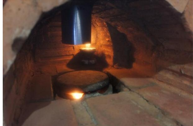
The oven chamber features the holey rocket stove beneath the oven floor, a clay disc to deflect the hot gases sideways and unto the walls of the oven, an extended metal cylinder at the chimney. The combination of the two deflectors (the disc and the cylinder) causes the heat to circulate inside the chamber thus give a more uniform and retained heat. My thanks go to Jon and Flip Anderson and Larry Winiarski for the lessons I gathered from their earth oven stove.
