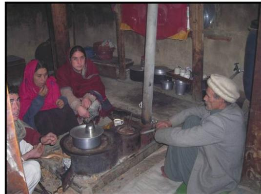
*BACIP model home with water warming facility (note blue tank in upper right and pipe inlet to stove).*
